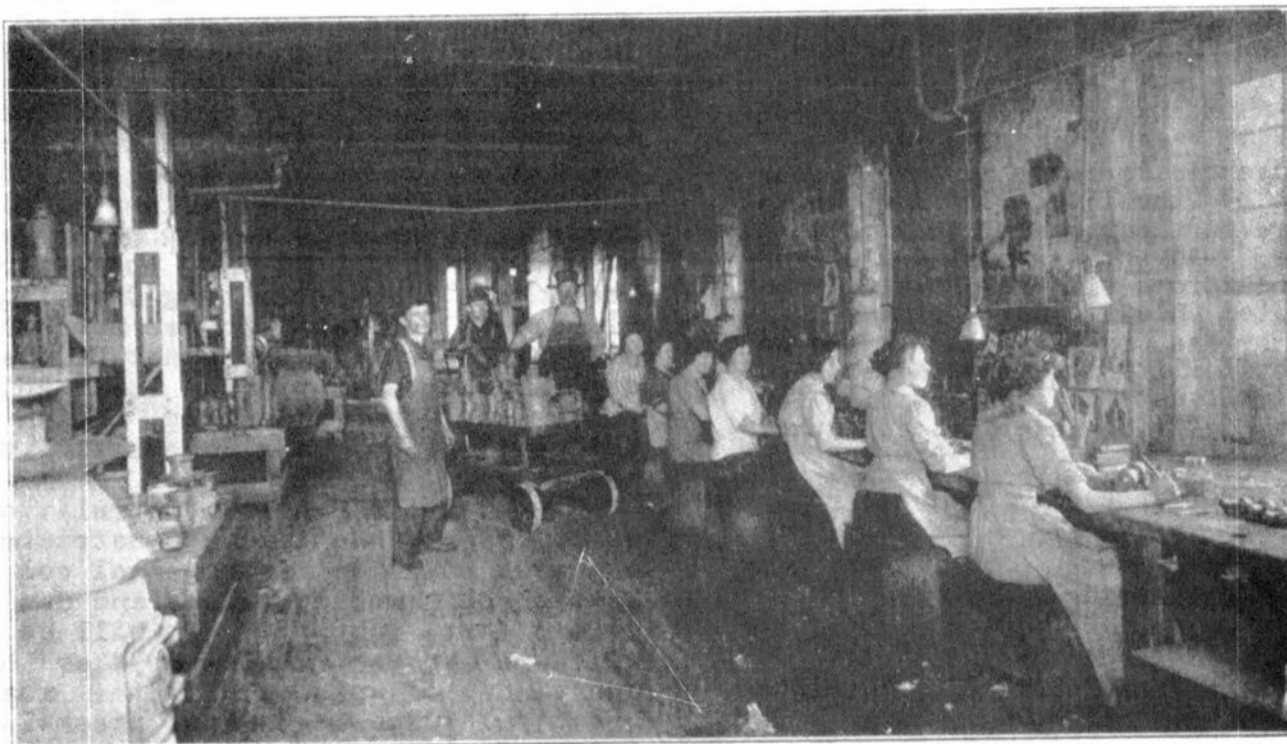
SECTION EAST—MOLD CLEANING DEPARTMENT To obtain high quality Glass highly polished molds are essential.
