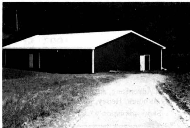
3200 Square Foot Storage Building Built in 1985 to House Molds, Tools, Memorabilia and Old Club Records
