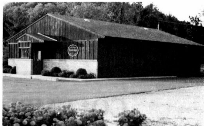
Museum Today After Renovation, Expansion and Reroofing
