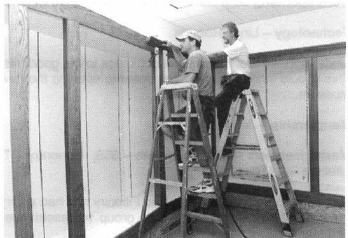
Dave Edwards (right) and Joe Endly (left) of Edwards Construction work on the crown moldings of the new showcases
