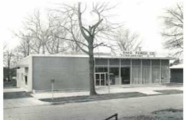
The completed building in 1966
